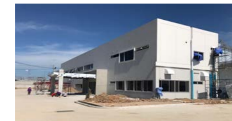
Coldstore +10 °C, Showa Industrial (Thailand) Co., Ltd.
