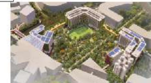
Singapore Institute of Technology (SIT) centralised campus in Punggol
